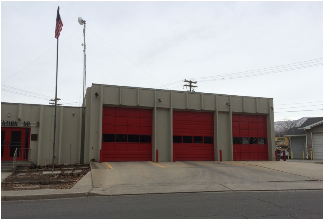
Current Sugar House Fire Station 3 located on Simpson Ave. near Fairmont Park
